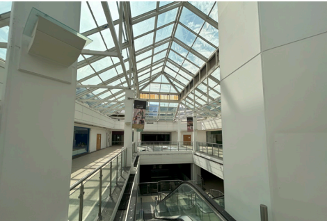
Fig 05 - Site Photo of Atrium
