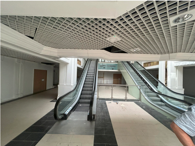
Fig 08 - Site Photo of Lower Atrium
