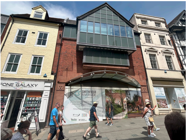
Fig 12 - Site Photo of Pride Hill Entrance
